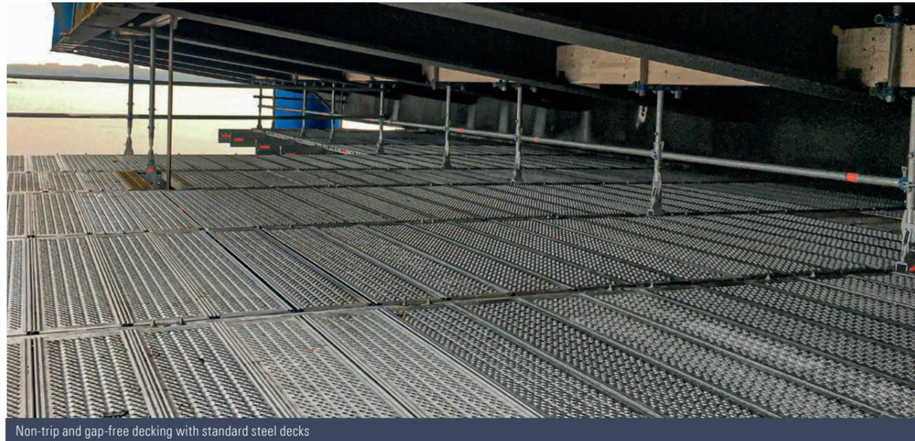
Non-trip and gap-free decking with standard steel decks
