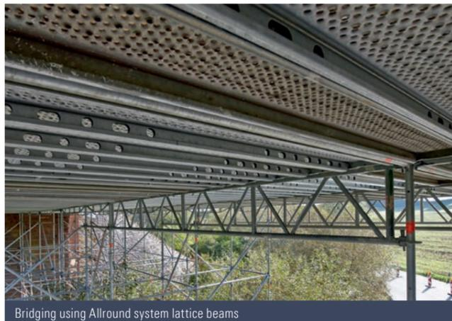
Bridging using Allround system lattice beams
