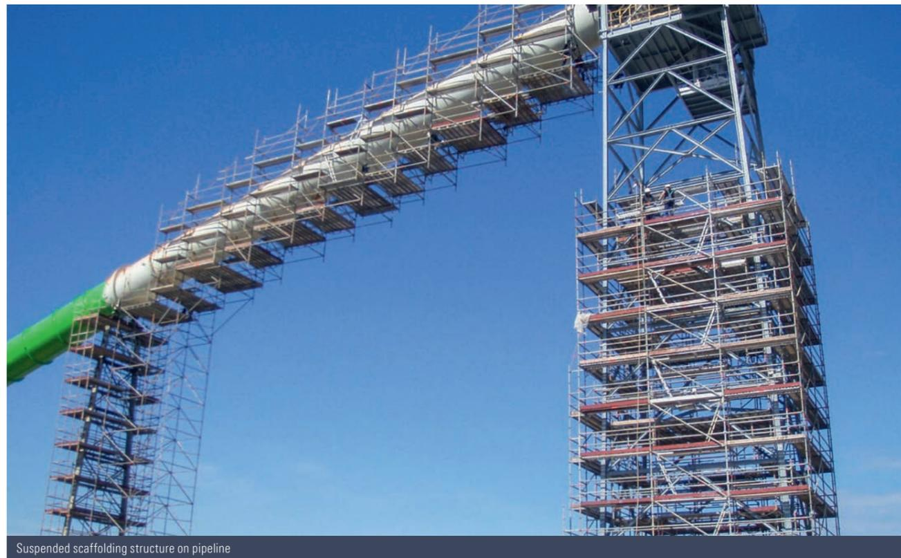
Suspended scaffolding structure on pipeline
