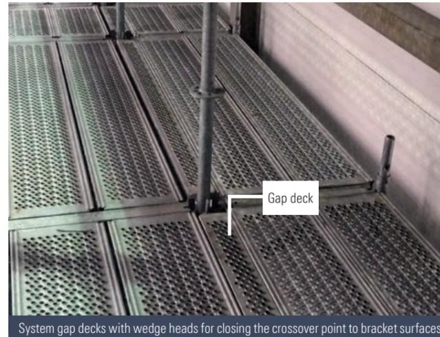
System gap decks with wedge heads for closing the crossover point to bracket surfaces
