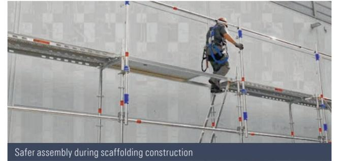
Safer assembly during scaffolding construction
