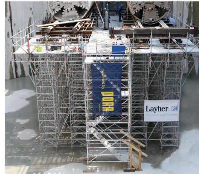
Load platform made of Allround Shoring TG 60 with integrated platform stairtower for setting down the drill heads
