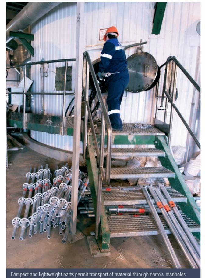
Compact and lightweight parts permit transport of material through narrow manholes
