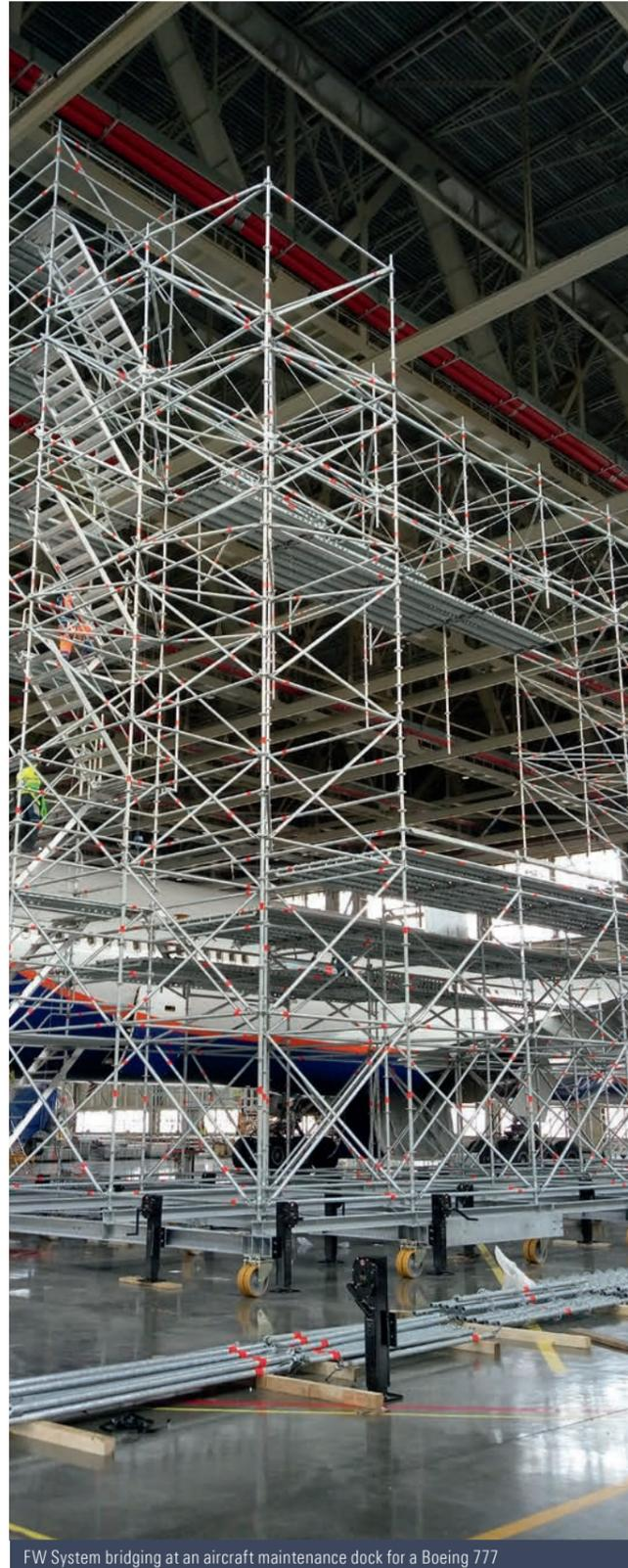
FW System bridging at an aircraft maintenance dock for a Boeing 777
