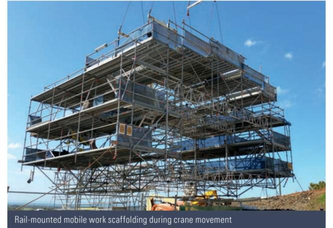
Rail-mounted mobile work scaffolding during crane movement
