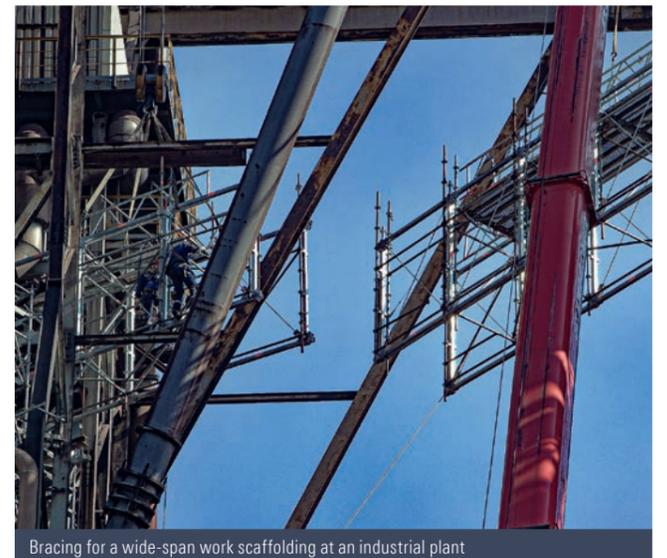
Bracing for a wide-span work scaffolding at an industrial plant
