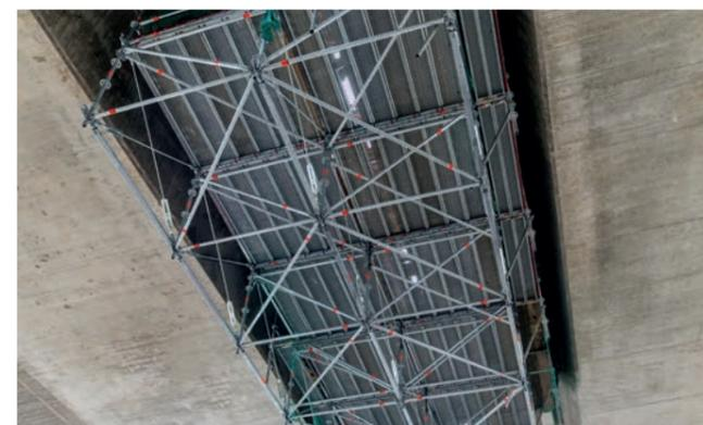
Mobile suspended work platform with Allround FW System
