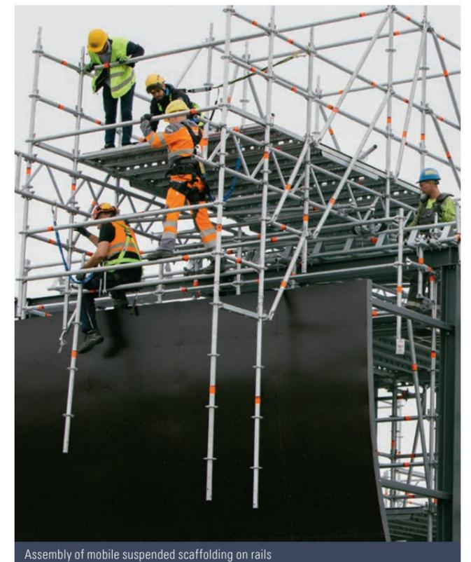
Assembly of mobile suspended scaffolding on rails
