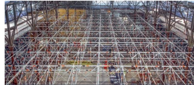
Birdcage scaffolding with Allround FW System inside a building – the floor area remains free, allowing normal work to continue
