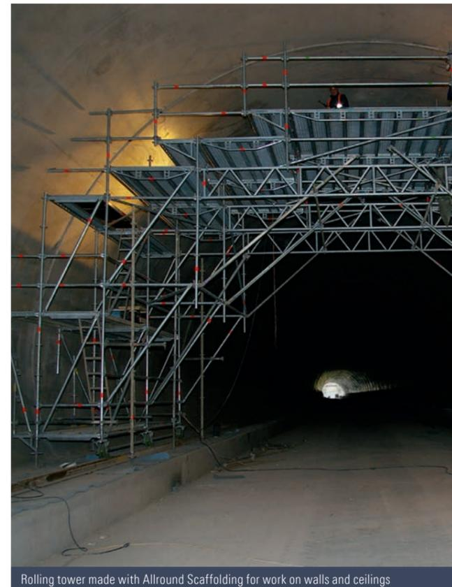
Rolling tower made with Allround Scaffolding for work on walls and ceilings
