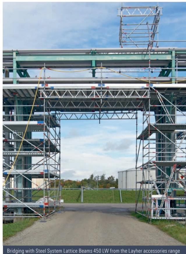
Bridging with Steel System Lattice Beams 450 LW from the Layher accessories range
