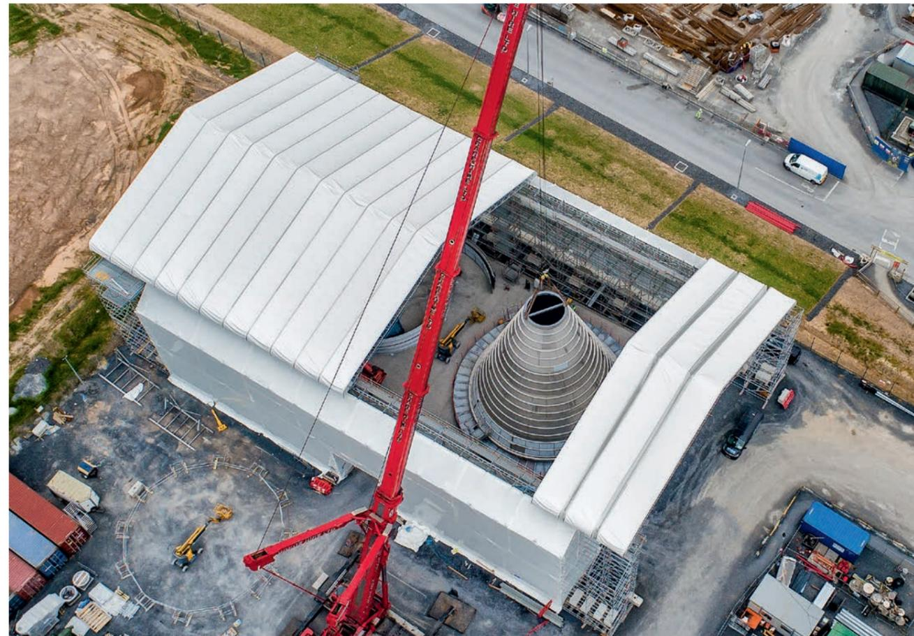
The roof of a temporary hall for assembling tanks independently of the weather was built using the Keder Roof XL from Layher in the reinforced bracing variant with a free span of 26 metres – and without a tie. This secured the clear height needed by the tanks. The substructure made from Layher's flexible Allround Scaffolding ensured an economical implementation of the site requirements, such as a walkway at the eaves level for moving the roof trusses – using standard components.
