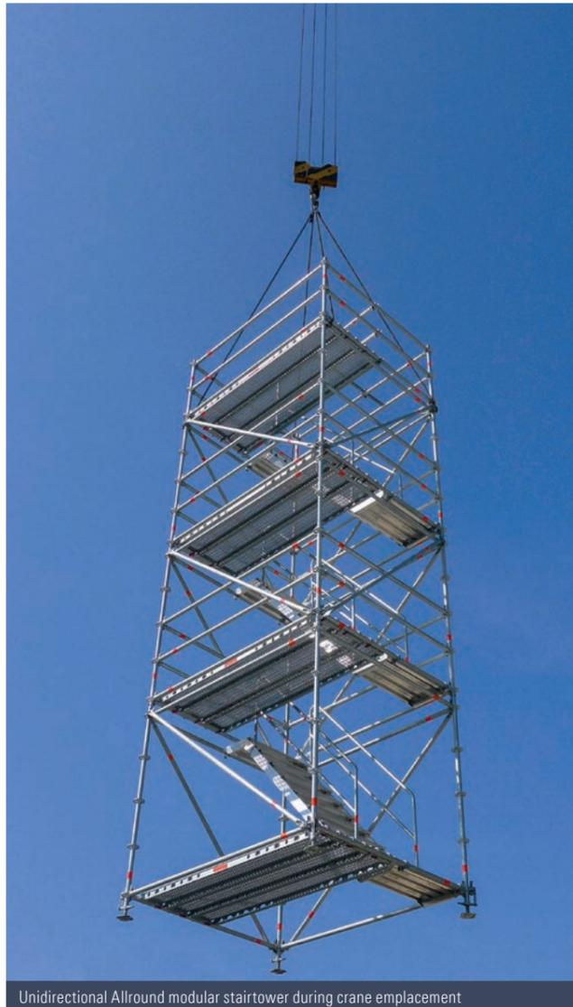
Unidirectional Allround modular stairtower during crane emplacement
