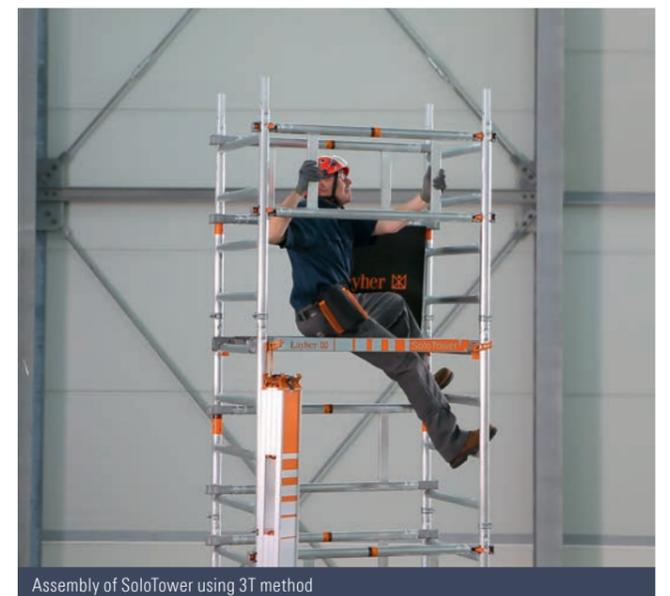
Assembly of SoloTower using 3T method
