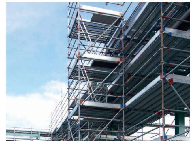
Internal ladder access with access decks
