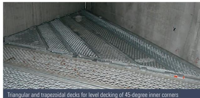
Triangular and trapezoidal decks for level decking of 45-degree inner corners
