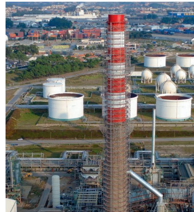
Circular scaffolding with Allround Scaffolding on a refinery column
