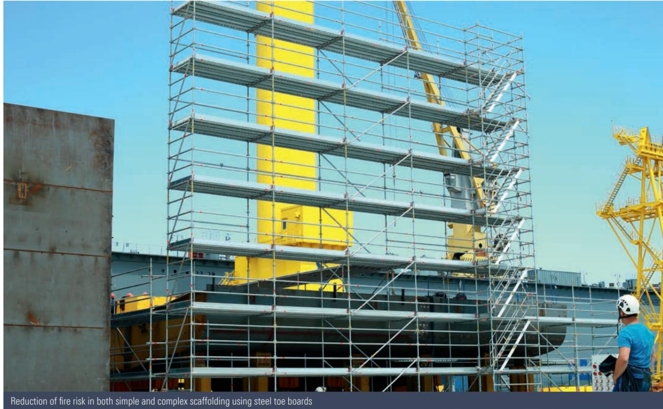
Reduction of fire risk in both simple and complex scaffolding using steel toe boards
