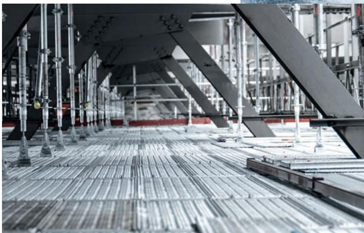
*The aluminium FlexBeams and Layher steel decks provided a quick and safe way to build the work platforms needed to refurbish the metal walkways.*
