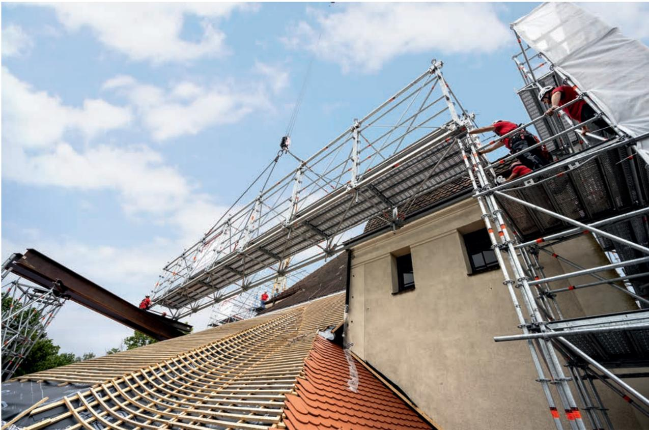
*Precision work by the truck-mounted crane as it places the Layher Allround Bridging System in position for bridging the roof area – and it's a perfect fit!*
