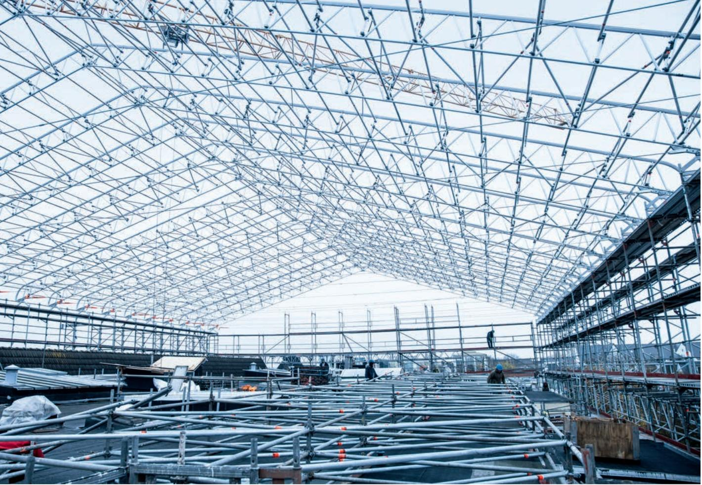
*More than 2,000 m<sup>2</sup> of Keder Roof XL were erected directly on the free-standing SpeedyScaf Scaffolding and three "scaffolding tables" hooked in.*
