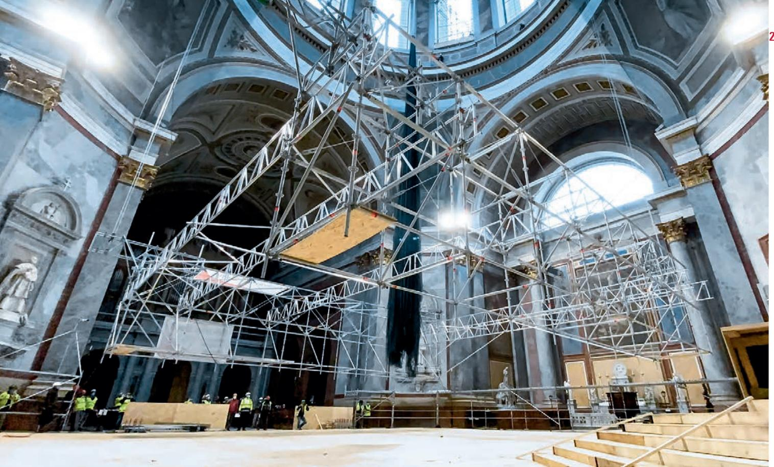
The lightweight access bridge was pre-assembled on the floor of the church, then lifted to a height of 34 m with winches and anchored there.
