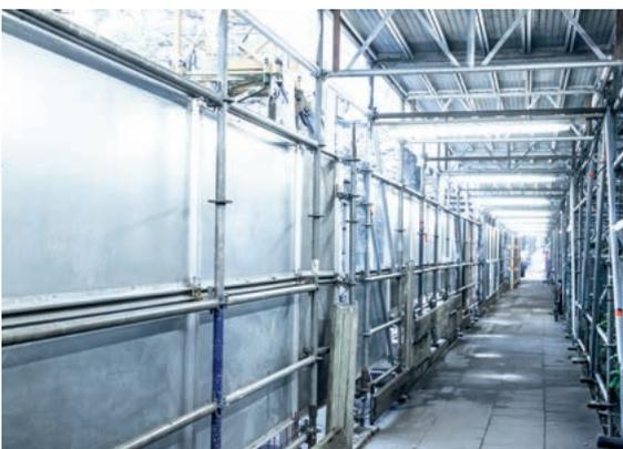
*Pedestrian tunnel made from Layher Allround Scaffolding and Protect System elements.*
