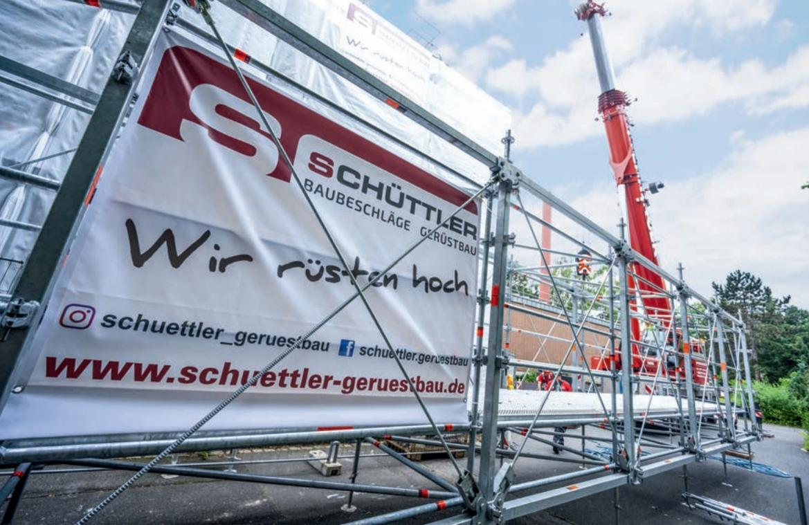
The Layher Allround Bridging System was preassembled safely on the ground before being moved by crane to the correct position in the scaffolding.
