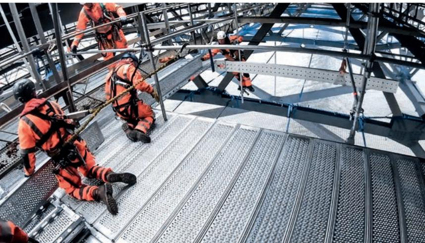
*The I-Scaff team were able to install twice as many m<sup>2</sup> per day with Layher's Integrated System as they were in earlier phases without the aluminium FlexBeam.*
