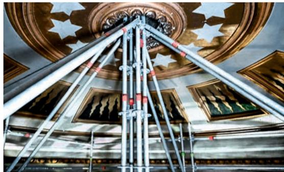
*The scaffolding for refurbishing the apex was suspended from the centre of the dome using Layher Allround material.*
