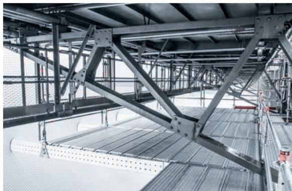
*The combination of aluminium FlexBeams and Layher system decks allowed amply dimensioned working areas with no major obstructions.*
