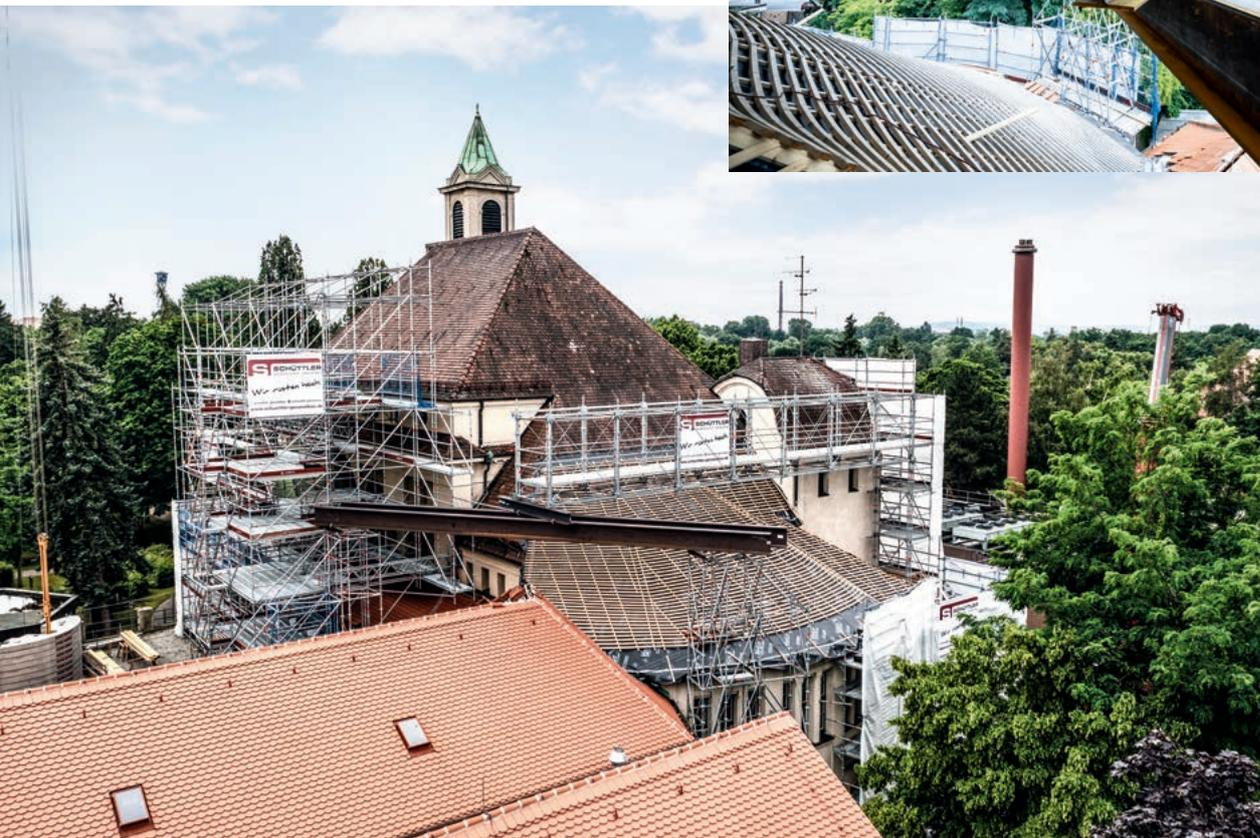
HEB 600 steel beams support the Layher Allround Bridging System.
