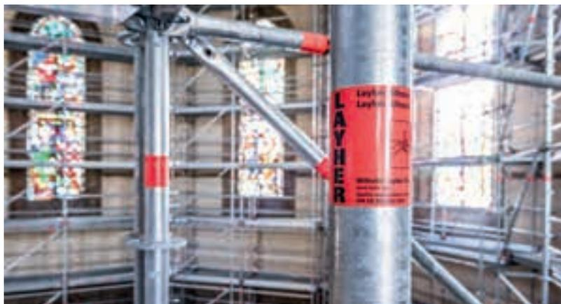
*The top walk-on scaffold platform at 37.50 m in height, just underneath the main nave, allows the craftsmen and restoration experts to safely access their vertiginous workplace.*
