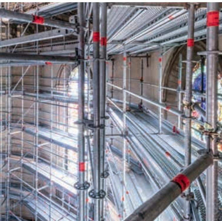
►► A Layher platform staintower provided safe access to the work platforms. The Layher platform stair makes safe and effortless ascent and material transportation possible without impairing the work area.
