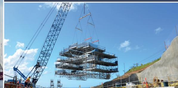
Crane-movable tunnel scaffolding | Tunnel repair
